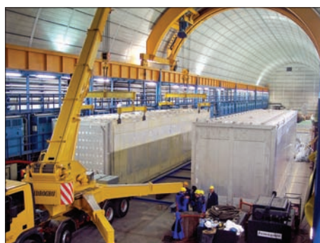
Fig. 6. The two half-module cryostats of ICARUS T600 just after they arrived in hall B at LNGS in December 2004. (Image credit: Francesco Arnedo LNGS-INFN.)
